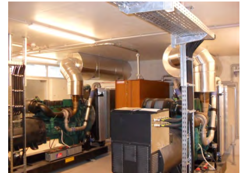
2 550 kVA parallel Amras Tunnel ASFINAG Tirol
